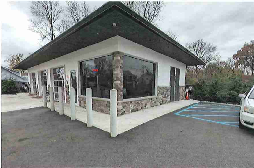
Existing walkway and bollards along the northeast side of the service bays and office.
