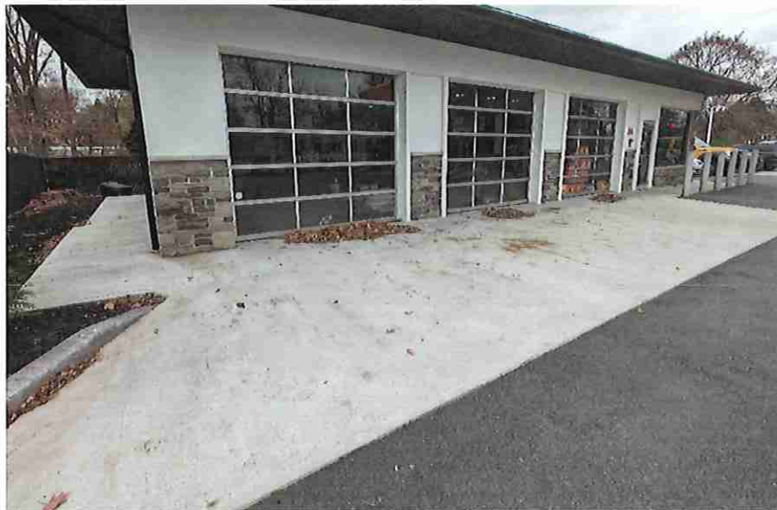
Concrete slab along service bay entrances. This may be saw cut or channelized with bollards to form a walkway.
