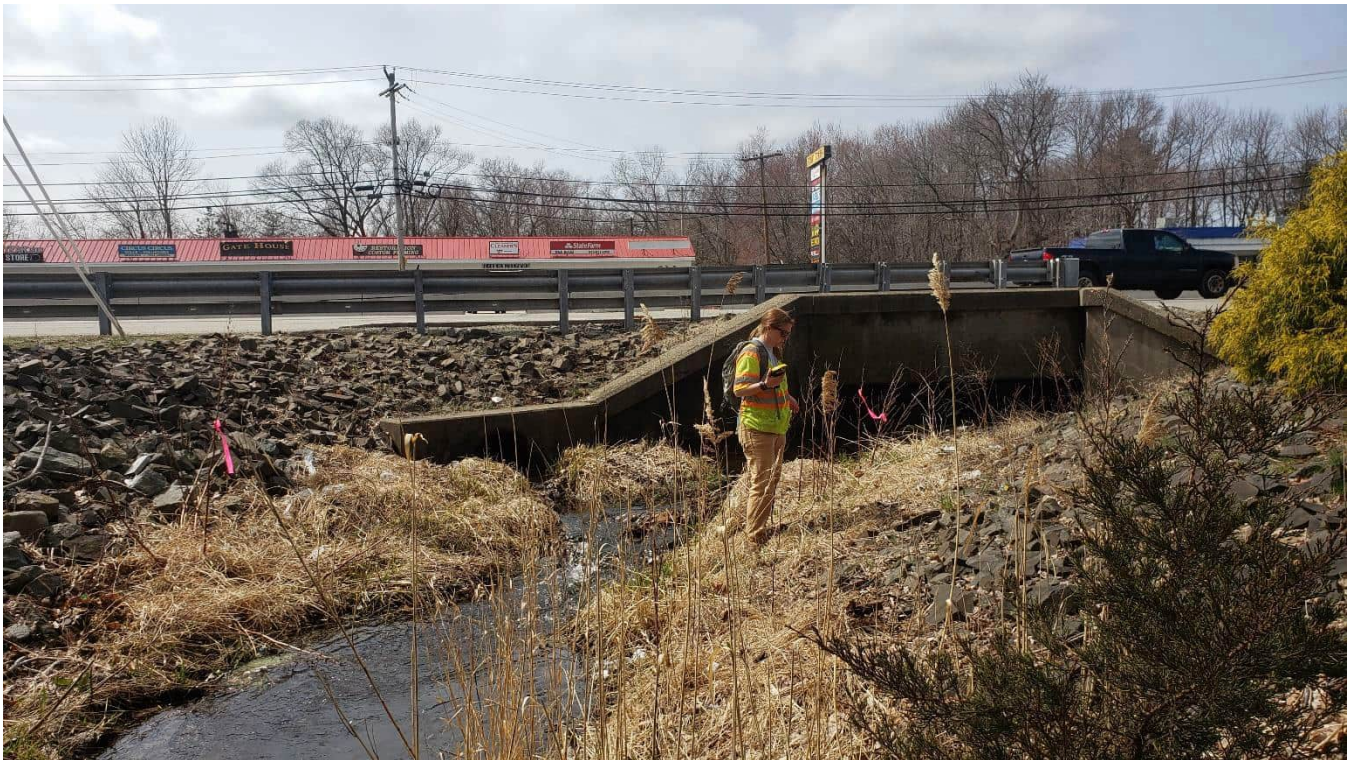
Photograph 64 – A view of Stream JBG-S upstream, facing northwest.
