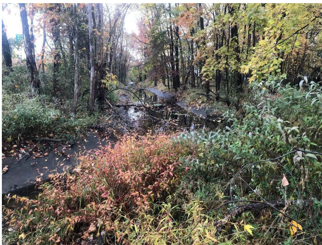
Photograph 108 – A view of Ditch DFJx-S/concrete ditch, facing northwest.
