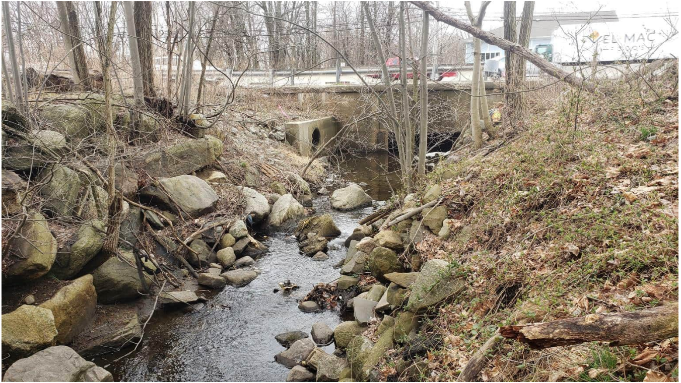
Photograph 61 – A view of Stream JBE-S upstream, facing west.
