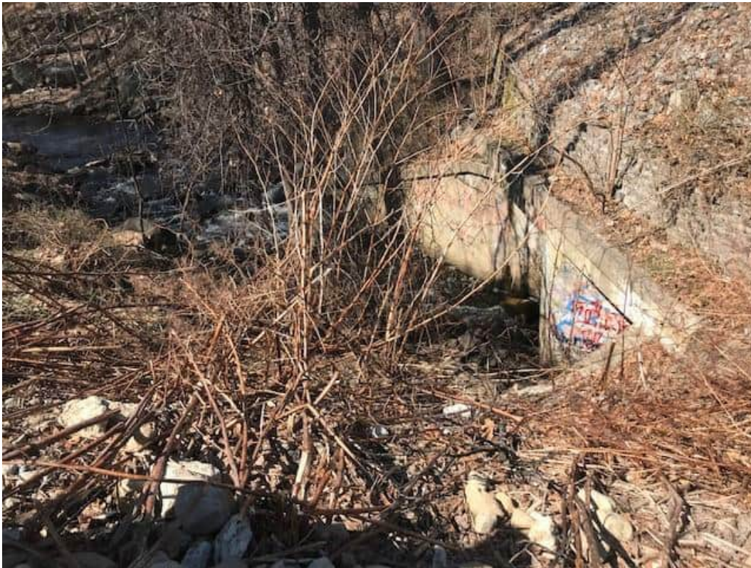
Photograph 28 – A view of Stone House Brook (DFZ-S) on the southbound side of Route 23, facing northwest.
