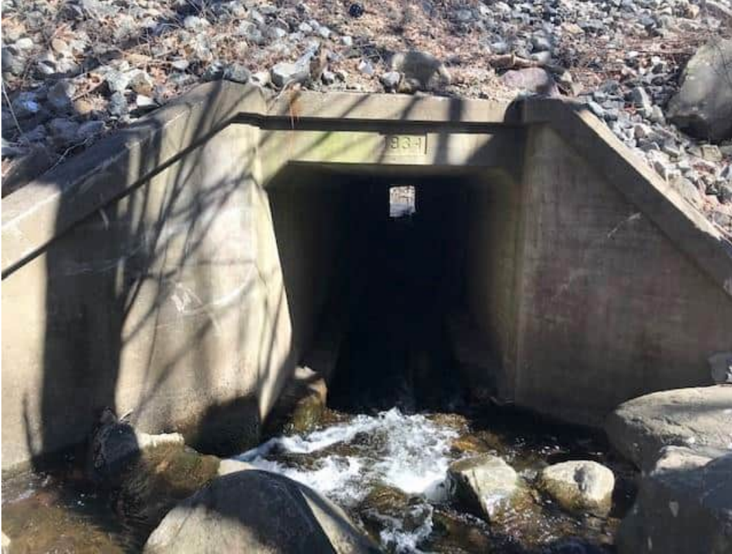
Photograph 9 – A view of Stream DFE-S downstream on the southbound side, facing north.
