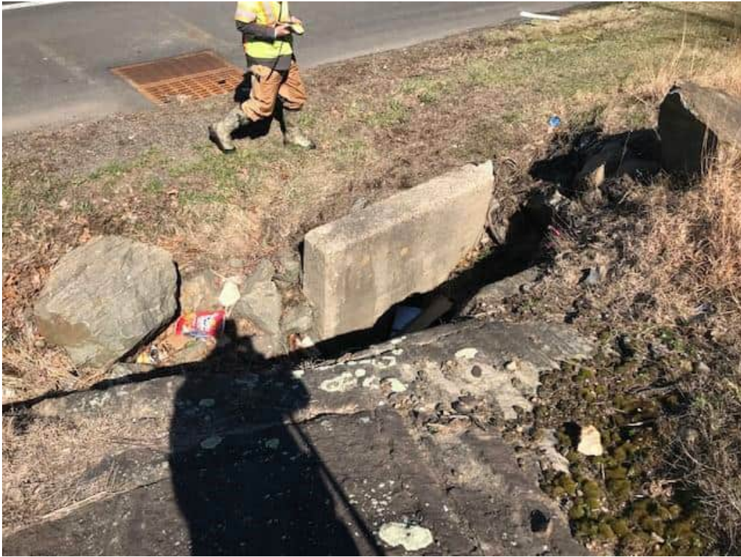
Photograph 25- A view of Stream DFN-S culvert and adjacent bedrock, facing northeast.
