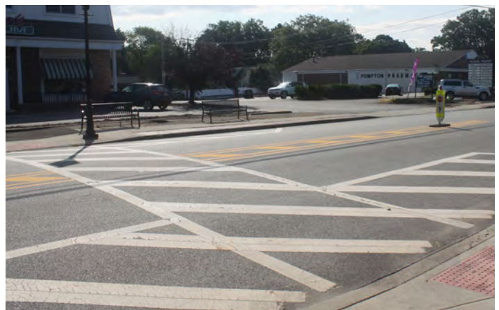
Example of painted curb extensions along Newark-Pompton Turnpike.
