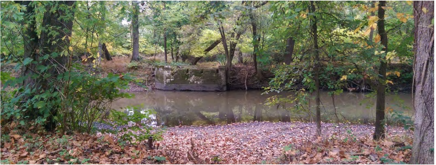
Photo of bridge abutment in Pompton Lakes, looking from Pequannock Township
